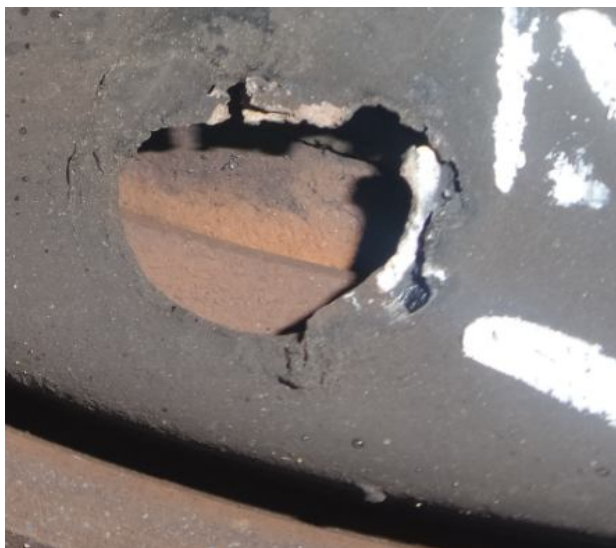
Axle 2 left – adequate linings
