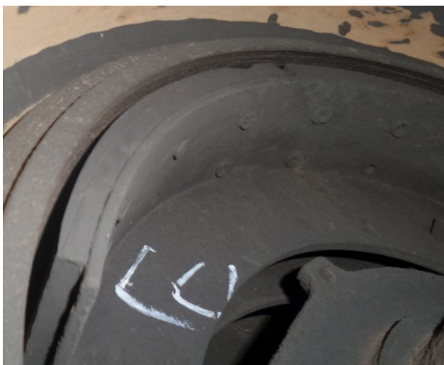
Axle 1 left – adequate linings
