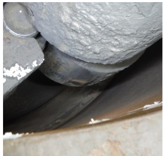
Axle 2 right – excessive roller marks
